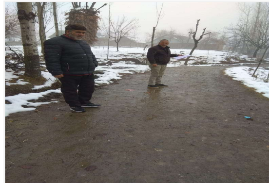
Construction of Road from Lachmanpora to Khan Mohalla Gujjarbasti Sitaharam
