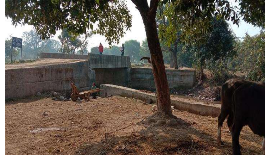
Constt. of culvert along with edge walls at Mirpur Jaggo to Gujjar Basti at Mirpur jaggo
