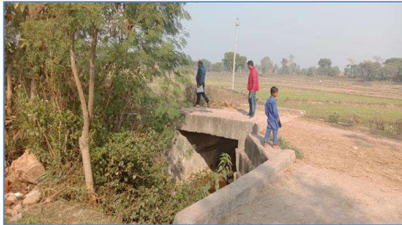
Constt. of culvert along with edge walls at Mirpur Jaggo to Gujjar Basti at Mirpur jaggo
