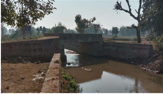
Constt. of culvert along with edge walls at Mirpur Jaggo to Gujjar Basti at Mirpur jaggo
